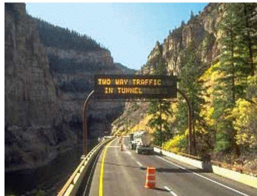
Hanging Lakes Tunnel, I-70, Colorado
