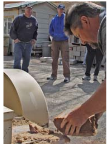
Construction Tech lecturer Rick Krouth demonstrates the adobe-making machine, which is powered on biodiesel this year.
