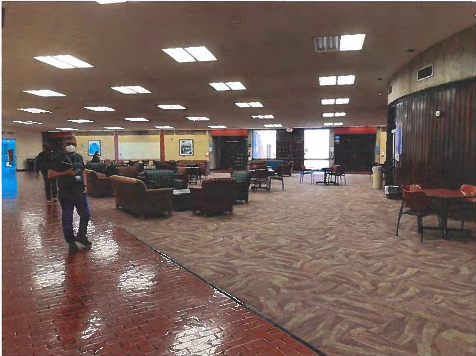
Existing Lobby Finishes with dated carpet and paint scheme. Paneling and doors from original construction in 1969.
