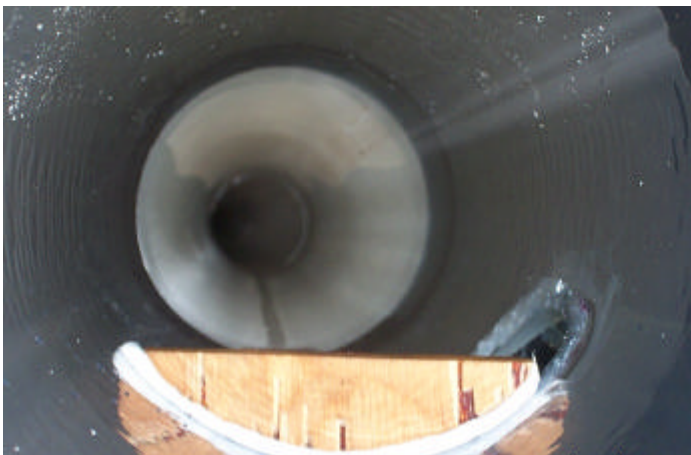
Photo 3. Low flow diversion curb
