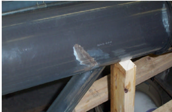
Photo 2. Low flow diversion alternative with diversion going below rather than the side of the pipe.
