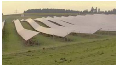
Solar installation near Munich
