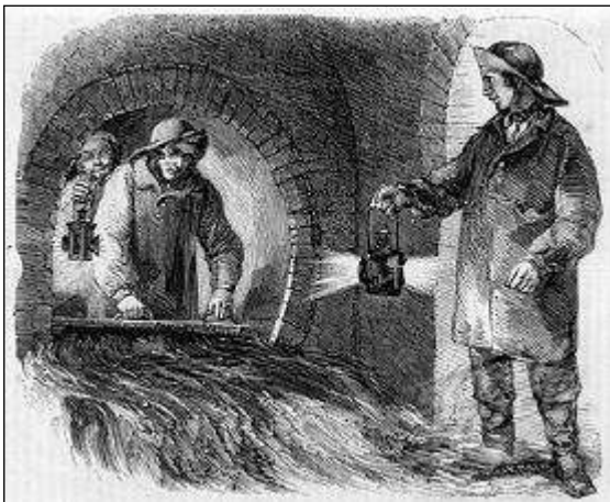
Flushing a London sewer, 1861
