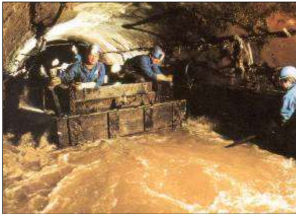
Hydraulic barge used for sewer maintenance, 1978.
