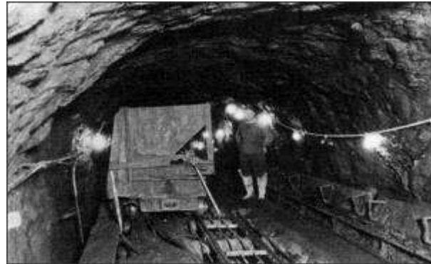
Construction prior to concrete lining.
