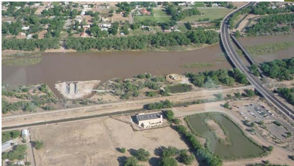
Diversion Dam & Pump Station
